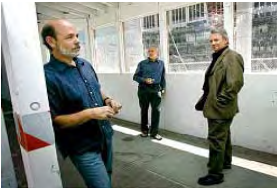
Stephen Goldsmith, John Schaefer and Gilberto Schaefer stand in front of a walkway window at a downtown demolition site, where they would like to turn the demolition of the malls into a museum. Kristin Nichols, Deseret Morning News
